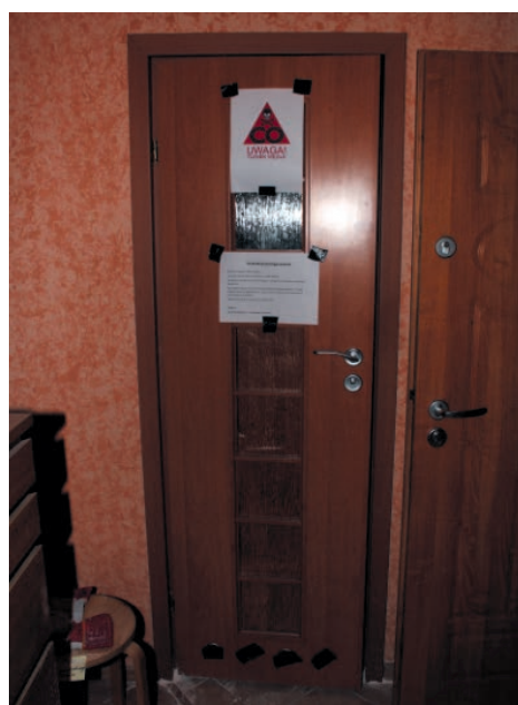
Fig. 2. Door with sealed ventilation openings and with chemical danger warnings stuck on.
